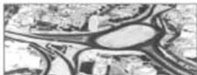
Msida multi-level intersection
